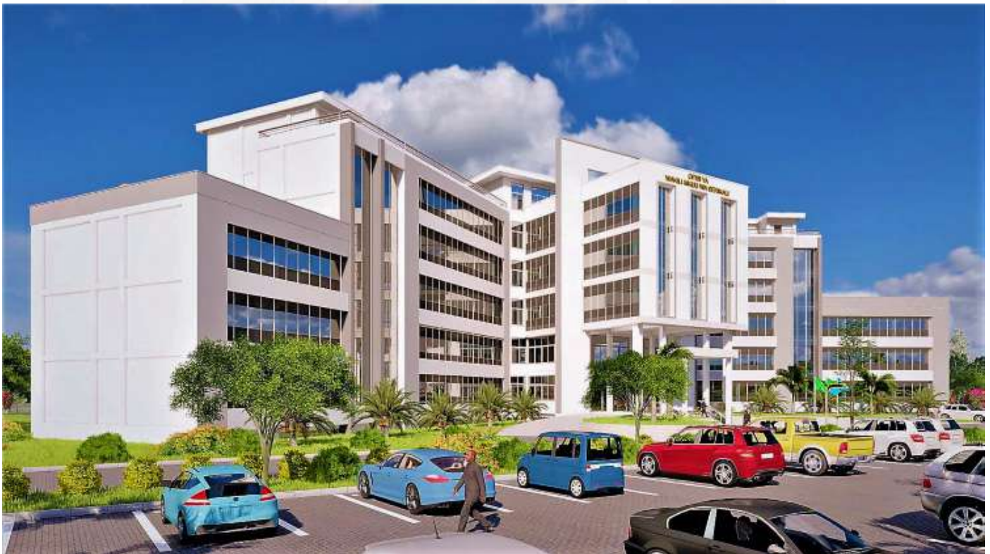
The side view of the new Solicitor General's Office building which is under construction within the Government City, Mtumba area in Dodoma region.
